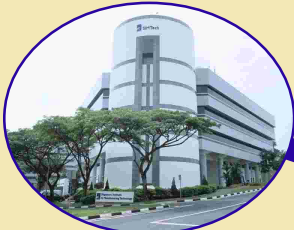
SIMTech Tower Block
